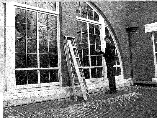
Rolfe de la Motte installing the window
