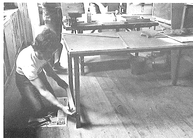
Geoff Pryor and his work bench and storage construction.
