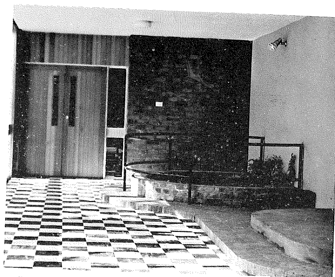
Convict well unearthed during construction. Now incorporated in foyer.
